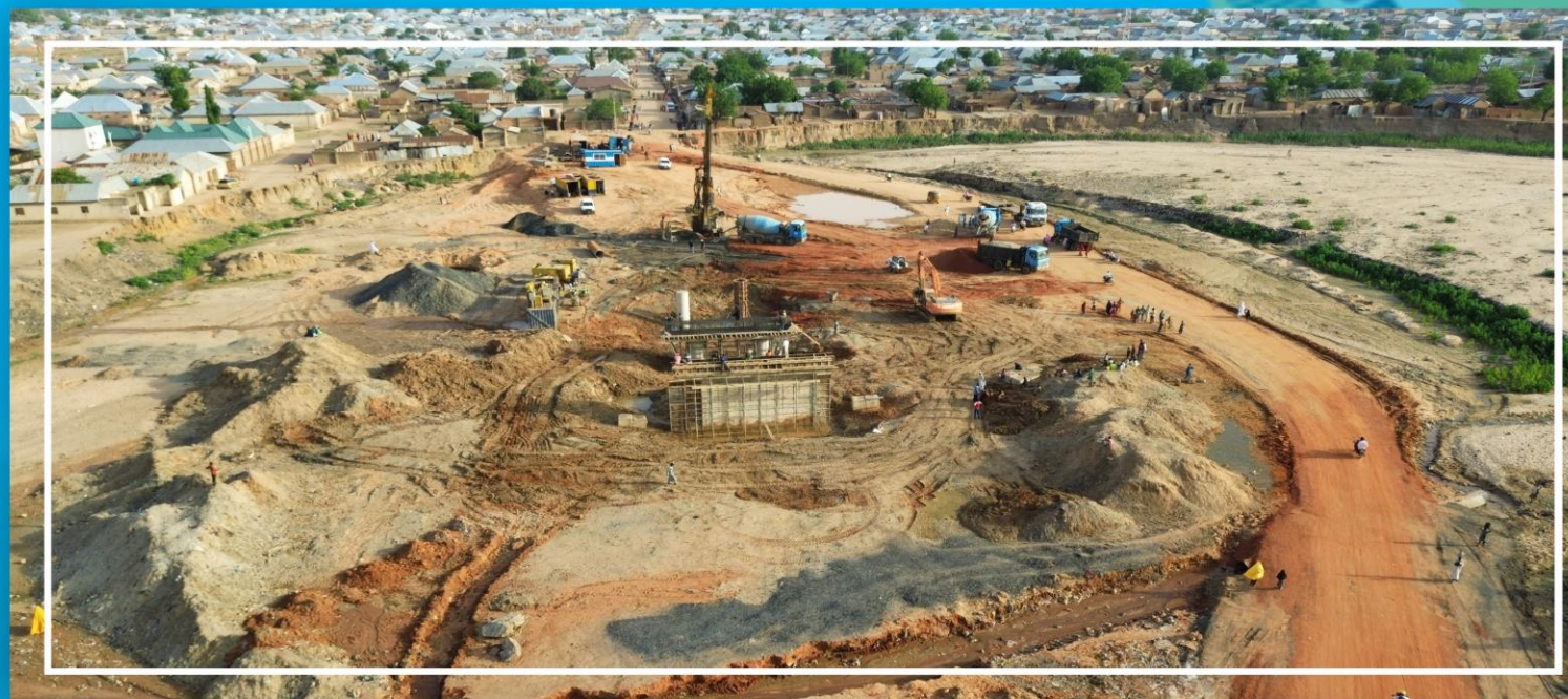
BRIDGE UNDER CONSTRUCTION AT HAYIN MISAU GOMBE
