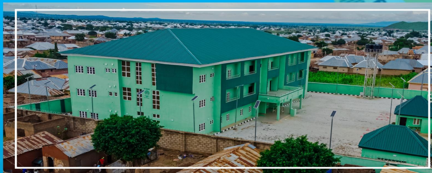
NEWLY CONSTRUCTED WOMEN AND CHILDREN HOSPITAL AT MALAM INNA GOMBE
