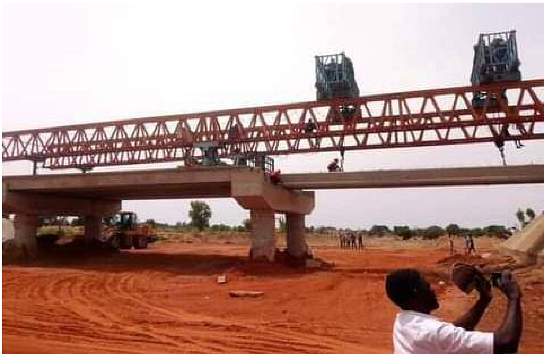
Bappar Bridge linking Funakaye – Dukku LGA
