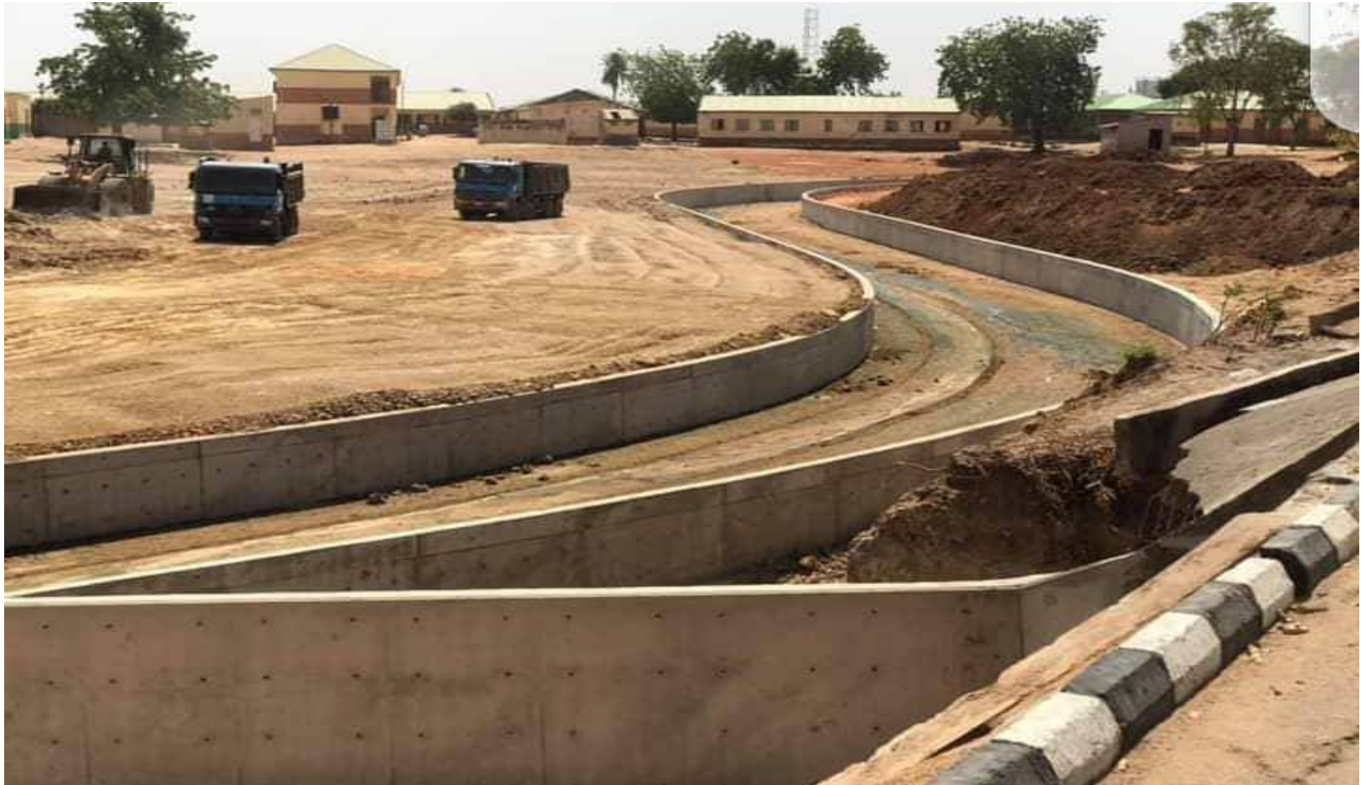
Gombe State University-Malam Inna Gully Erosion Control Project
