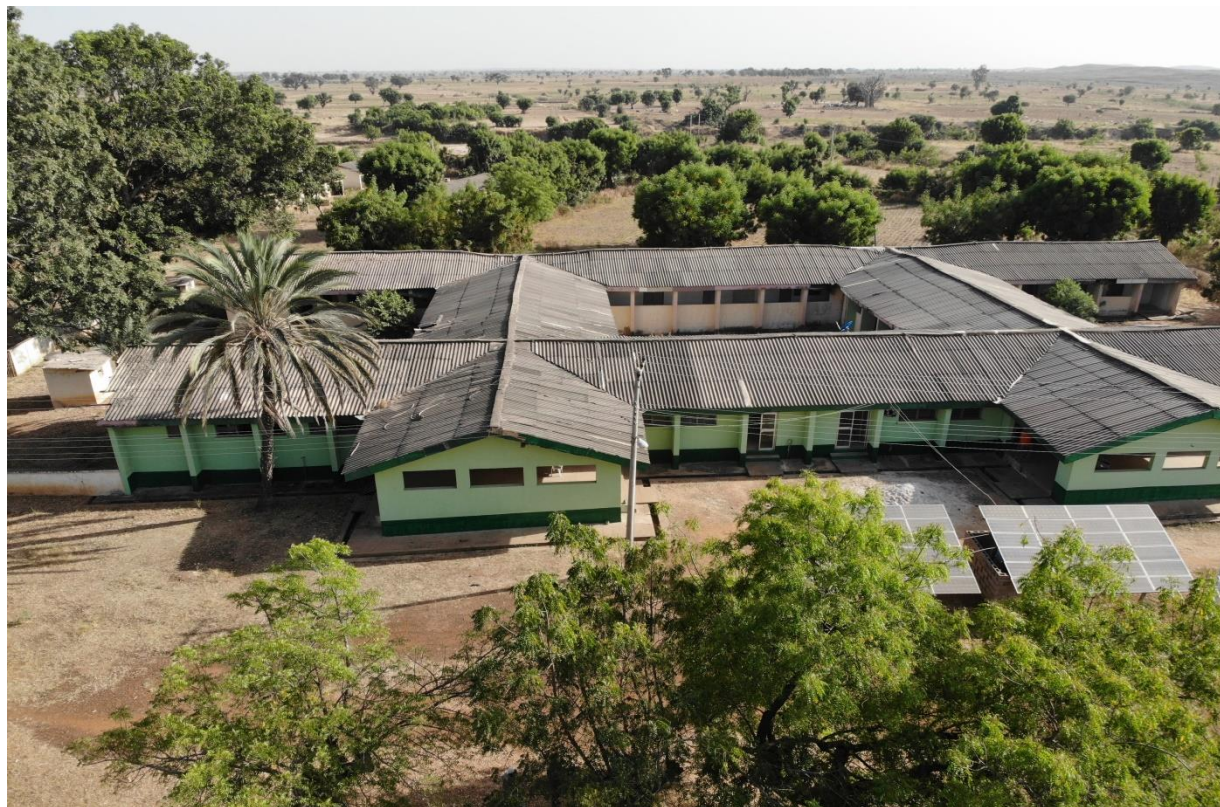
COTTAGE HOSPITAL KALSHINGI AKKO LGA (BEFORE)
